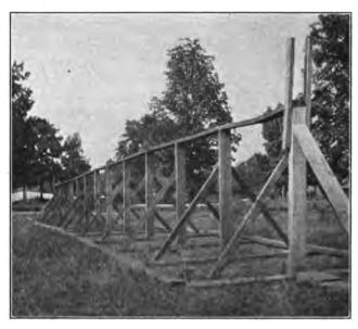
Fig. 91.—Pole framework used to dry yellow poplar, basswood, and cottonwood before placing it in a stuck pile.
